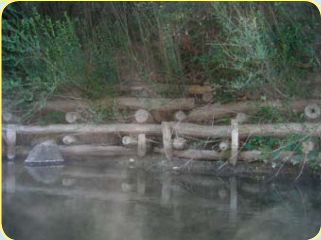
Figure 48 - Log matrix used to armor bank
