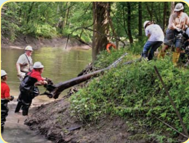
Figure 39 - Remove cut logs at designated place, above bankfull channel
