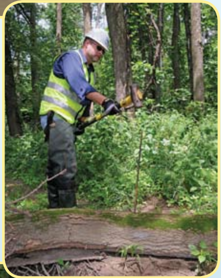
Figure 32 - Anchoring log to bank with rebar
