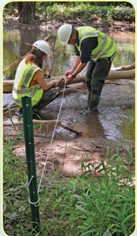
Figure 50 - Anchoring a log using the Palmiter Method
