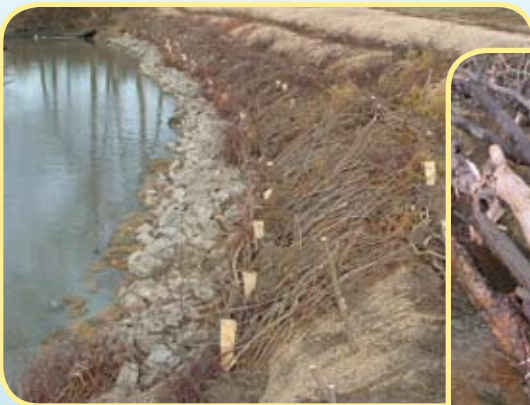
Figure 55 - Woody debris and rip rap combined to armor a streambank
