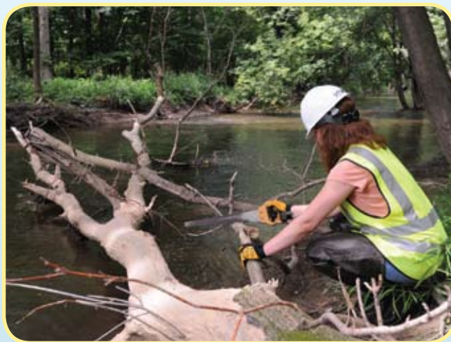
Figure 10 - Using hand tools for LWD maintenance
