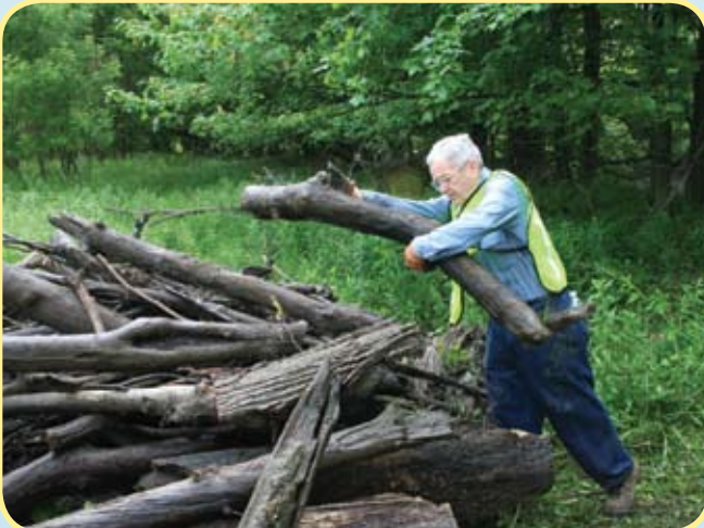
Figure 22 - Placing cut debris above bankfull channel
