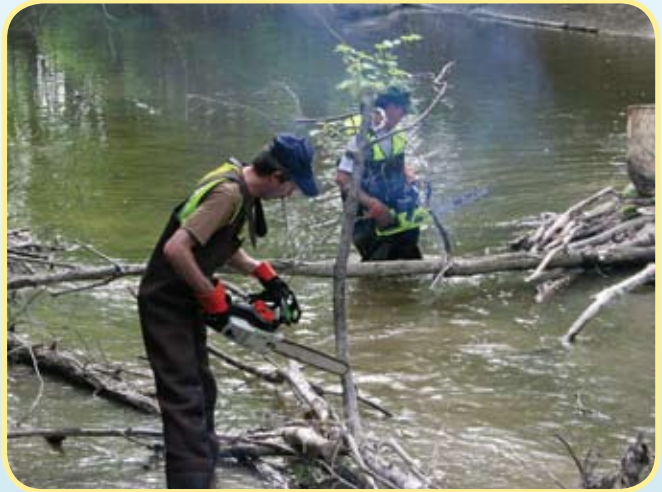
Figure 22 - Placing cut debris above bankfull channel
