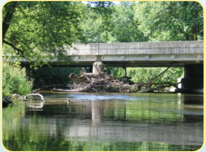
Figure 42 - LWD blocking culvert
