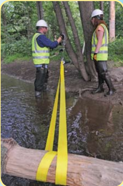
Figure 29 - Using a come-along to reposition log
