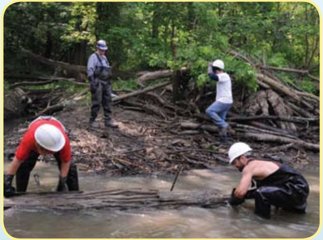
Figure 39 - Remove cut logs at designated place, above bankfull channel
