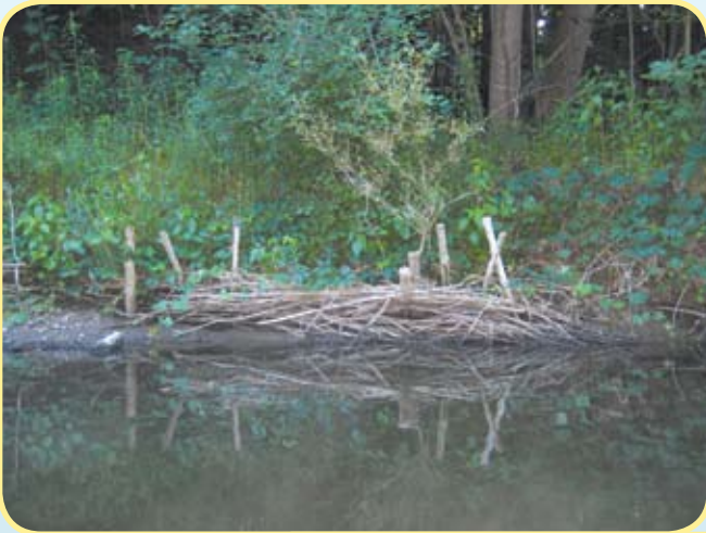
Figure 48 - Log matrix used to armor bank
