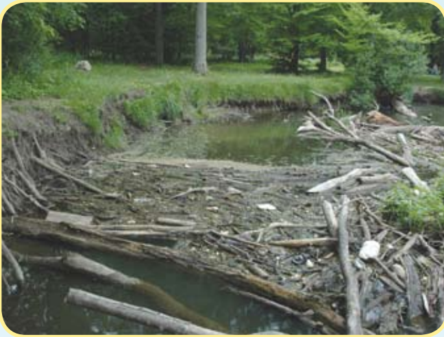
Figure 34 - A floating debris dam
