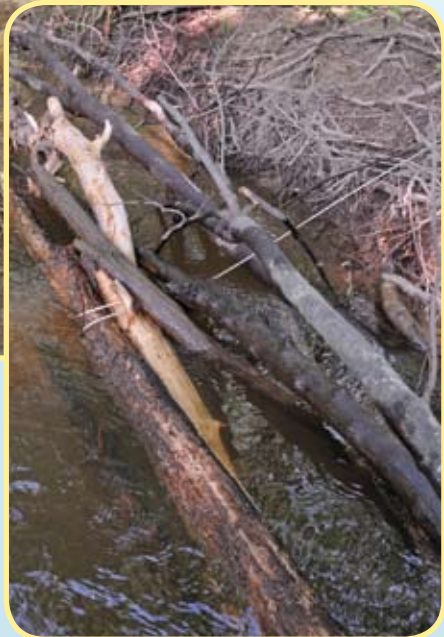
Figure 56 - Logs cabled together to armor eroding bank
