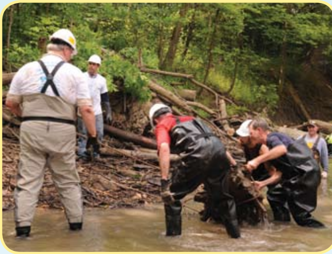
Figure 51 - Logs removed from a jam may be re-used to create habitat structures
