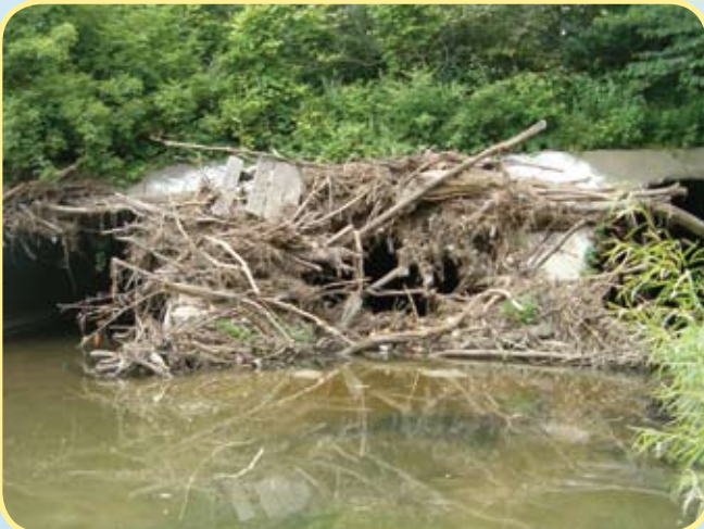
Figure 42 - LWD blocking culvert
